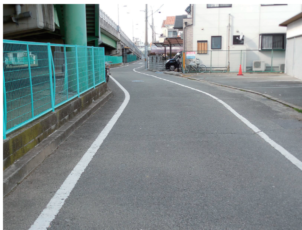
Fig. 1. Street where sewerage manhole cover was found in Amagasaki City, Hyôgo Prefecture, Japan.
