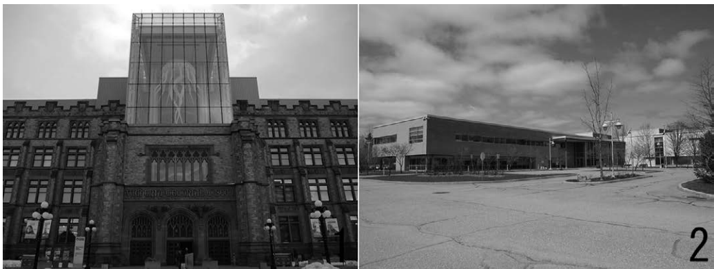
Figs. 1, 2. Canadian Museum of Nature. 1, Victoria Memorial Museum Building (Exhibitions & Programs), Ottawa, Ontario. 2, Natural Heritage Building (Administration, Collection & Research Divisions), Gatineau, Quebec.
