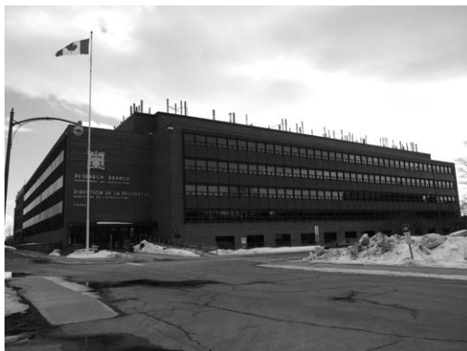
Fig. 15. K.W. Neatby Building, Ottawa.
