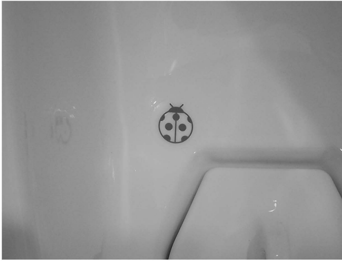
Fig. 2. Ladybug-shaped urinal target to reduce splashing as an aim to maintain hygiene in gentlemen's toilet.
